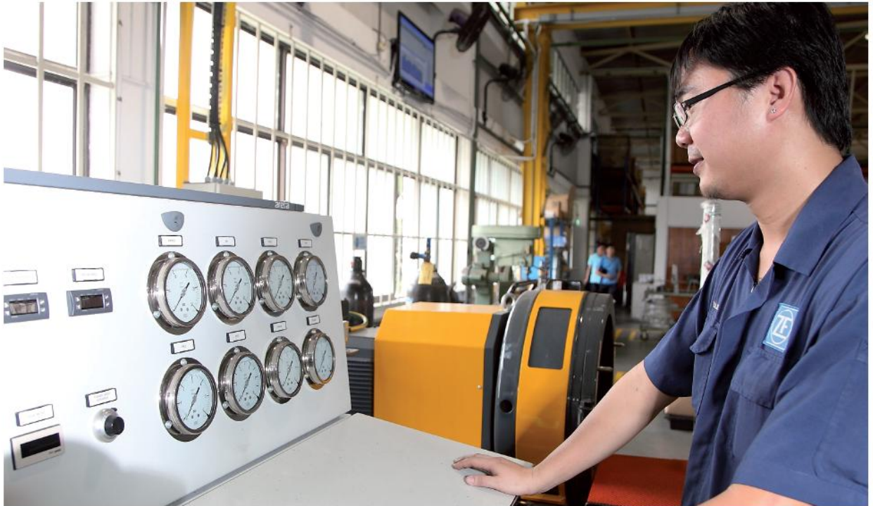
In Singapore, ZF has a 24/7 maintenance and service agreement with Port of Singapore Authority International.
